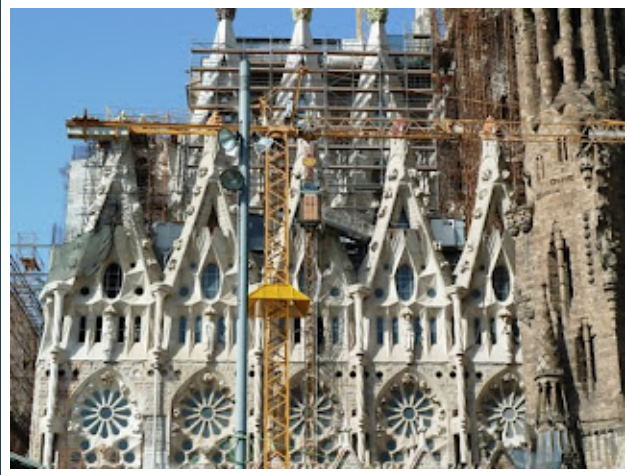
new section under construction
