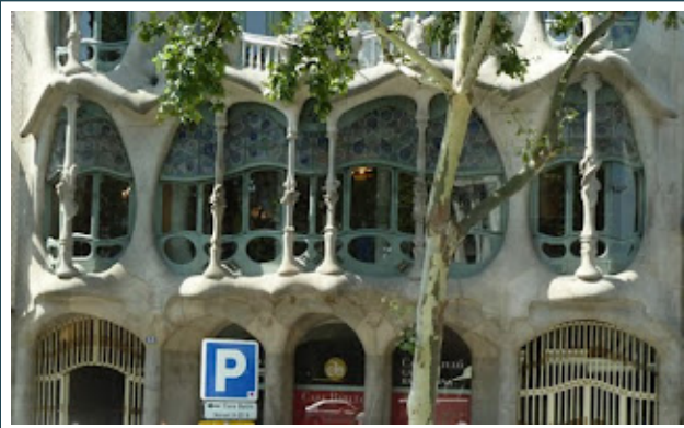
a Gaudi designed apartment building
